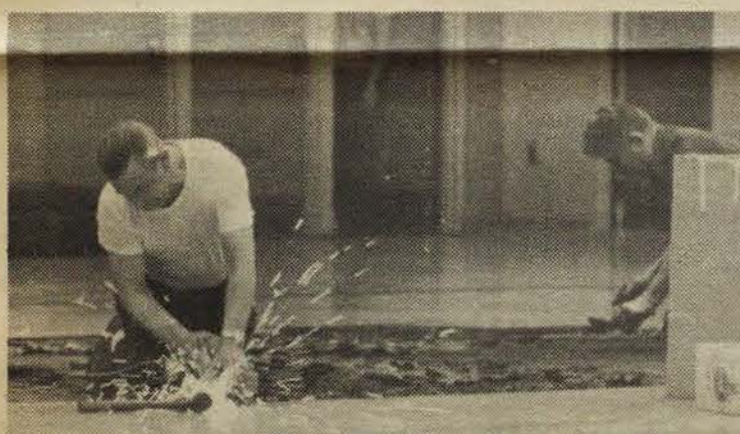
Sparks fly as workmen labor to repair the gym floor. A broken water pipe over the holidays caused the floor to buckle.
