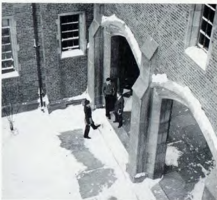
Outside of Chemistry
