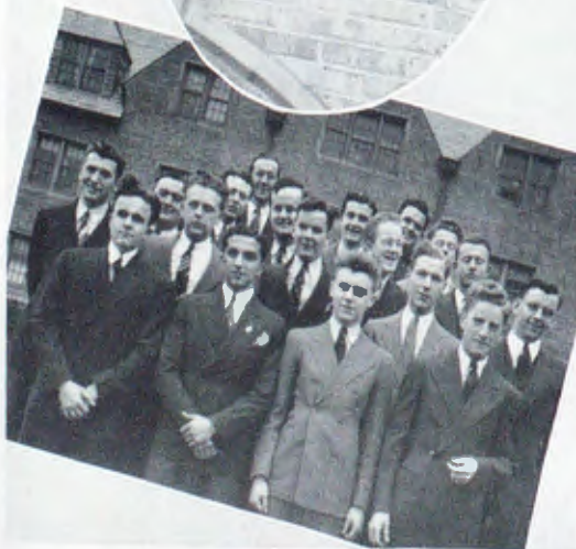
The Dormitory Servers
